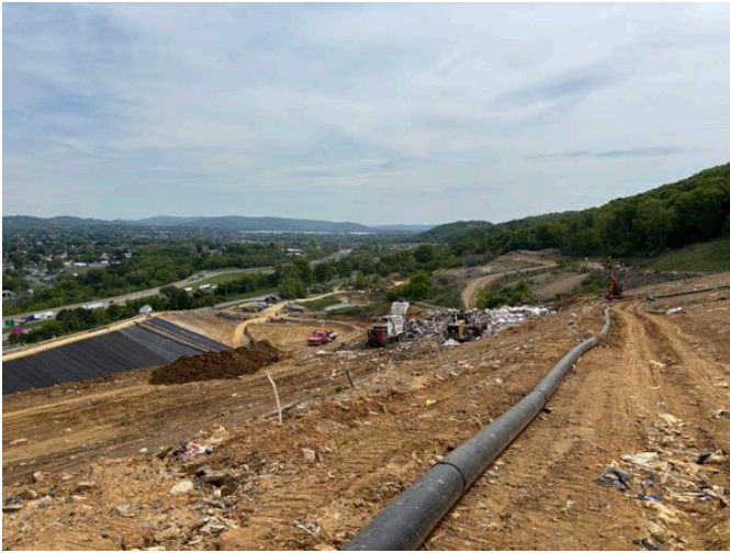
Photo #1: Working face in stage 7. Liner installation in stage 10.
