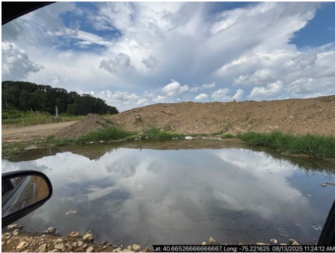
Photo #1: Pool of sitting water at exit of working face.
