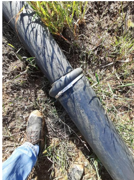
Photo 4: Nick in header pipe at GW-145.
