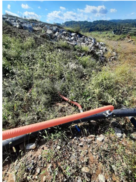
Photo 3: Low point in condensate line at GW-202.
