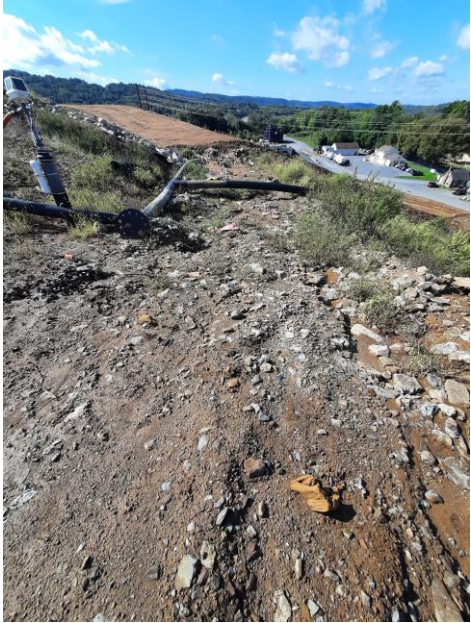
Photo 5: Some washout and erosion in 3E bench.
