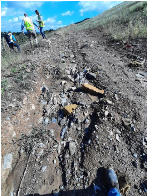
Photo 6: Some washout erosion and flagging in 3E bench.
