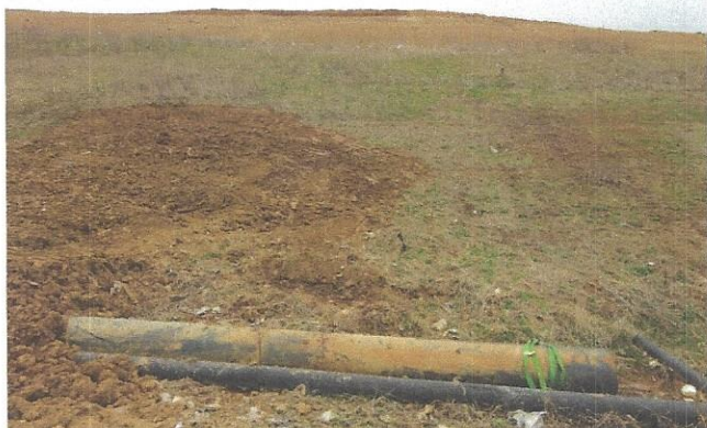
Photo 5: Leachate seep repair on northern slope just east of the candlestick flare.
