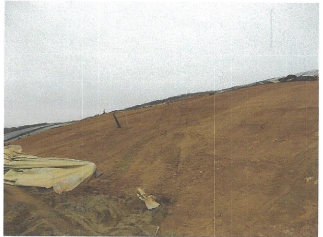
Photo 3: Wind damaged temporary cap on northern slope.
