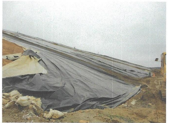
Photo 4: Repairs to far panel of temporary cap on northern slope.
