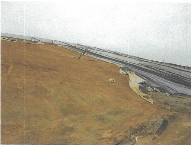
Photo 2: Wind damaged temporary cap on northern slope.
