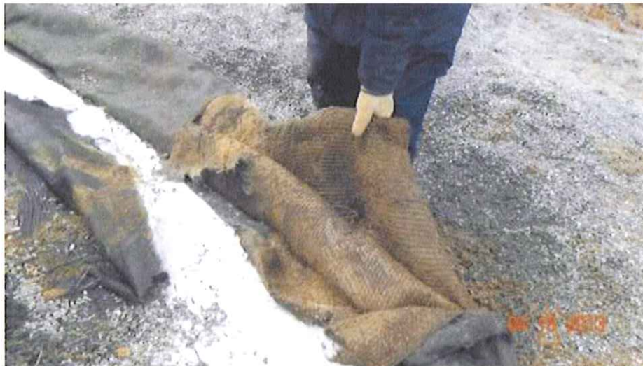
Figure B-2: Post-Slide Geosynthetics
