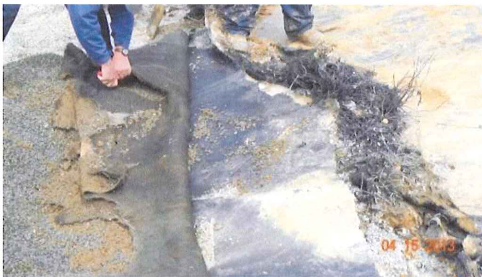
Figure B-2: Post-Slide Geosynthetics
