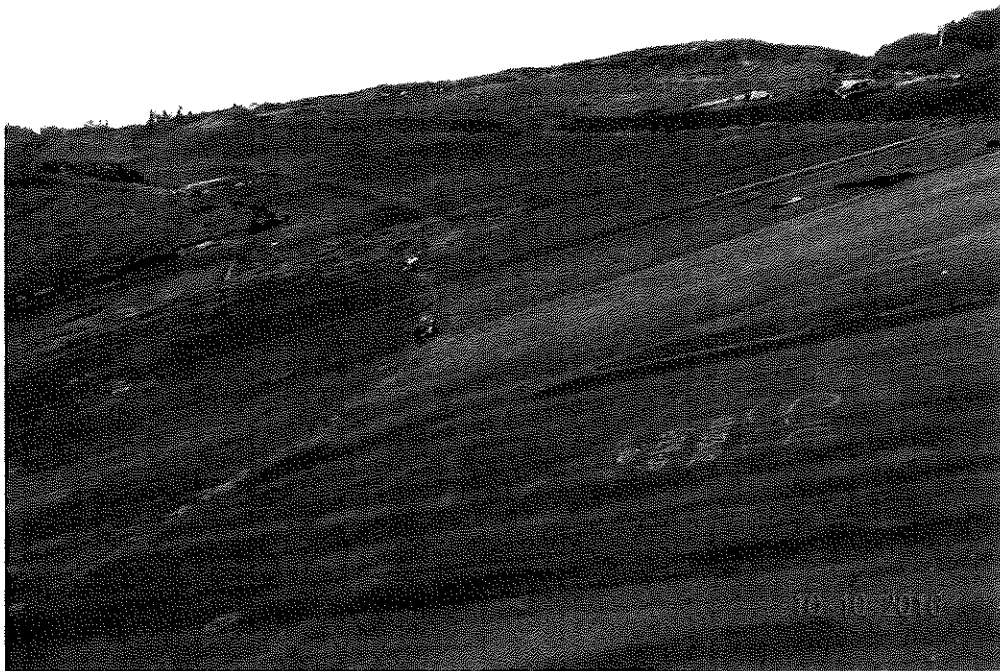
Figure B-10: Photograph of secondary geomembrane still present and intact on the slope in Stage 3E and a portion of Stage 3D.
