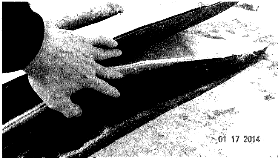
Figure B-9: Cross-section of liner system in slope failure area and photograph of liner system components after waste excavation.
