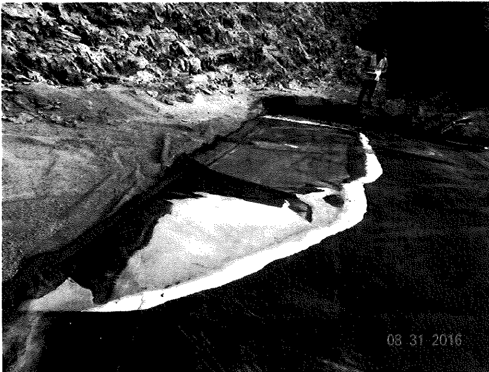
Figure B-15: Photograph of primary geomembrane/GCL interface interface movement.
