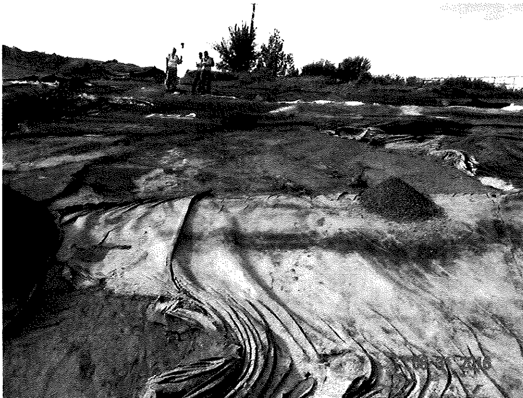
Figure B-13: Photograph of secondary geomembrane/compacted clayey subgrade interface movement.
