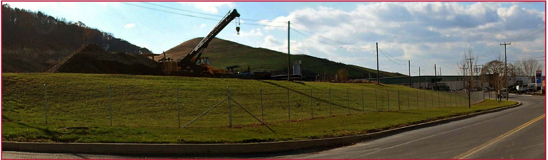
EXISTING LANDSCAPE - PHOTOGRAPH LOOKING WEST - INDUSTRIAL DRIVE
